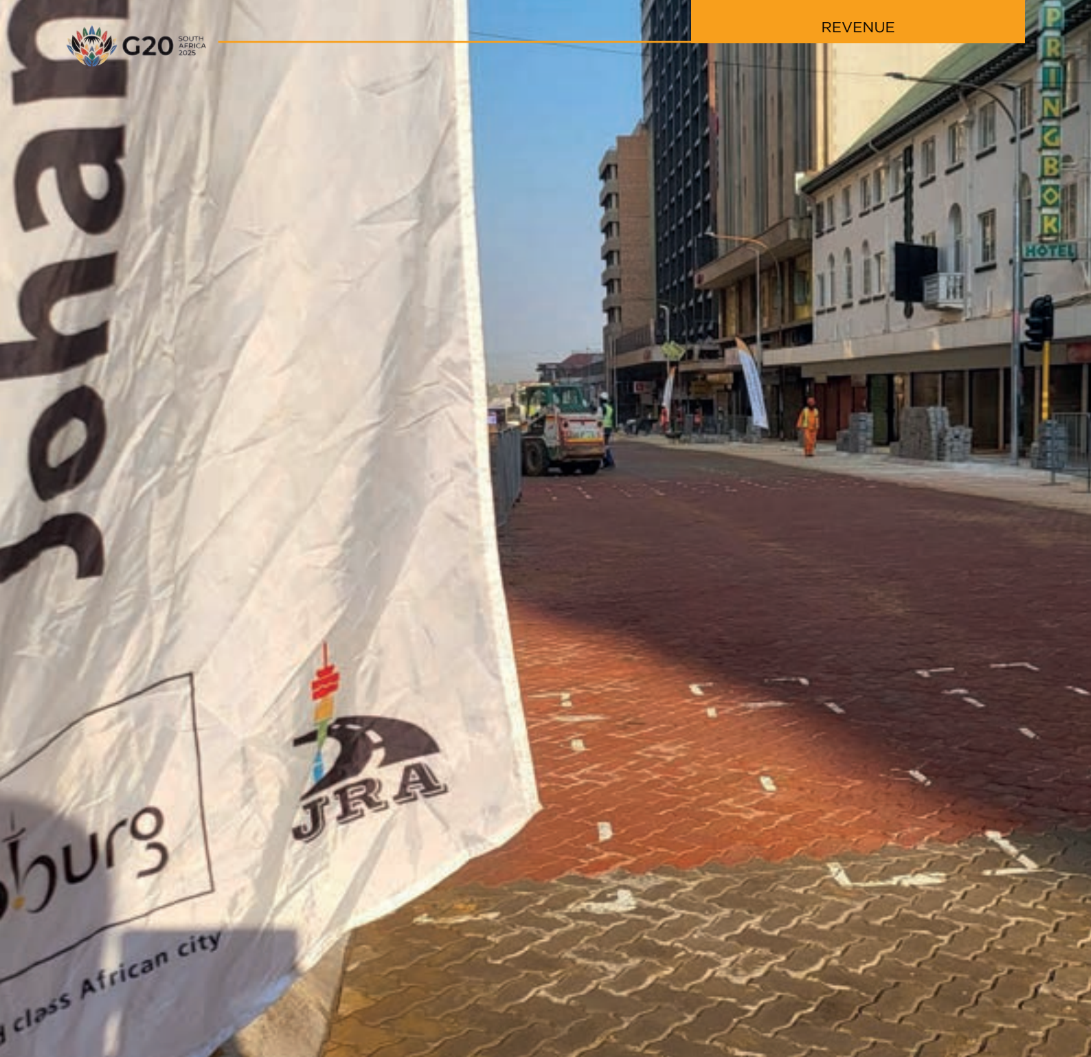
Lillian Ngoyi Street Repairs: Supplied
